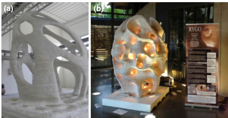
Fig. 19 a Radiolaria Pavilion: Andrea Morgante, founder of Shiro Studio, has collaborated with D-Shape to produce the Radiolaria pavilion, a complex, free-form structure produced using the world’s largest 3D printer. This rendering’s external measurements are 3×3×3 m and are a prototype for a final 10-m-tall pavilion to be built in Pontedera, Italy. “The structure is made of an artificial sandstone material and does not feature any internal reinforcement.” ( https://www.dezeen.com/2009/06/22/radiolaria-pavilion-by-shiro-studio/#more-33059 ). b While somewhat smaller, Bathsheba Grossman’s seven foot high “Cement” was also printed with D-Shape and was put on display in Vancouver, British Columbia, Canada. ( https://bathsheba.com/gallery/commissions/rygo/ ). Since 2014, it has been on display at the Gropps Gallery. It is a mathematical surface known as a gyroid
